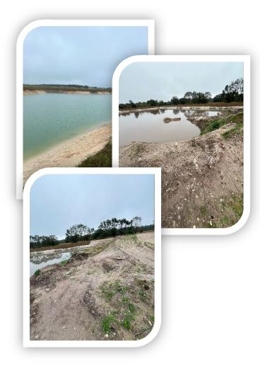
The stormwater ponds on tracts D3 and D4E in Ranches South have seen heavy erosion.
